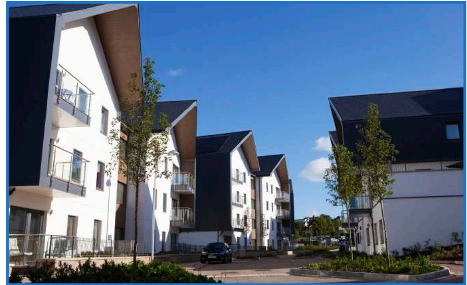
New housing development, Beechfield View, Torquay
